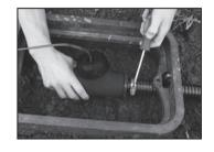
When using PVC, glue pipe into Slip Fitting using PVC glue (not included). Follow the glue manufacturer's directions for proper plumbing steps.
